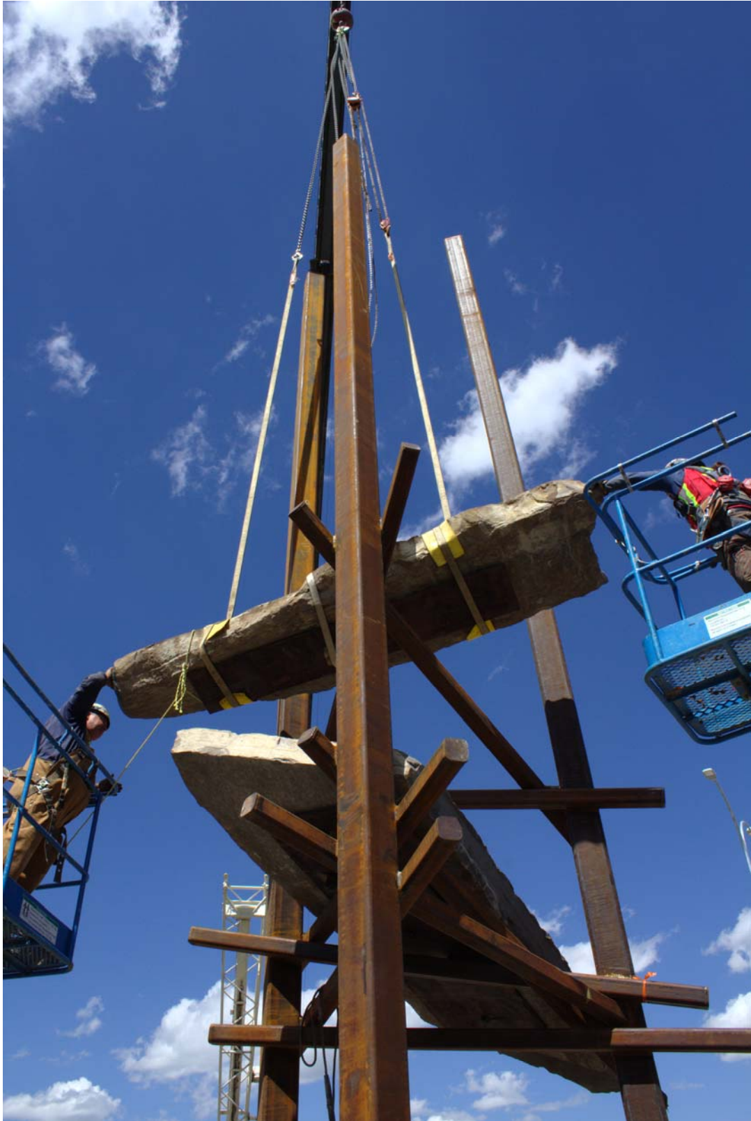
Figure 11. Triassic Towers, installation, 2017
