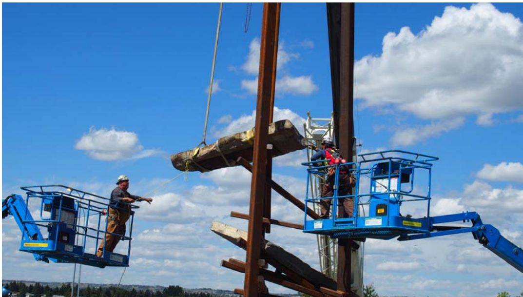
Figure 9. Triassic Towers, Installation, 2017.
