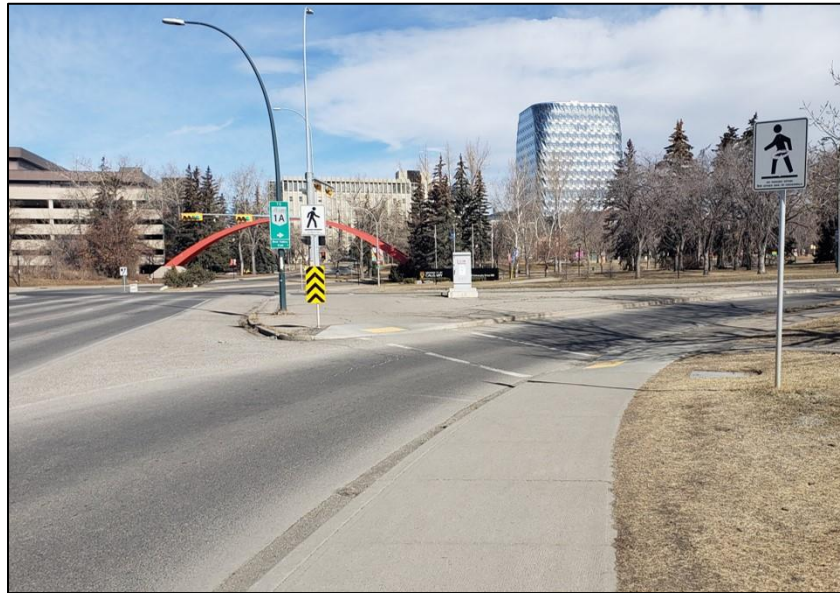
Figure 17. A slip lane is a road feature designed to avoid vehicle stoppages at right turns.
