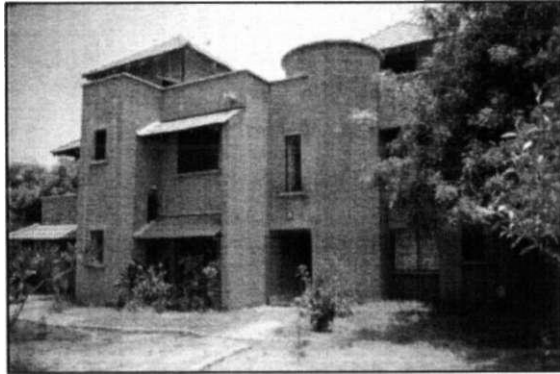
Figure 5.4: A group housing in Auroville. Compressed earth blocks were used for all pillars and walls with five per cent cement content. Local Terracotta tiles were used for roofing. Source: Iyer, S. (1997, October). Earthy pleasures . Indian Architect & Builder, 11 (2), 31
