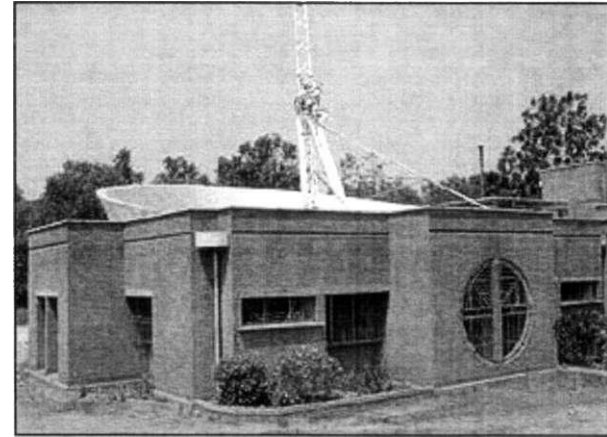
Figure 5.5: One of the community kitchens in Auroville that utilises solar energy for cooking. Source: AUT (1996c). The Solar Kitchen . Available at http://www.auroville.org/society/solarkitchen.htm
