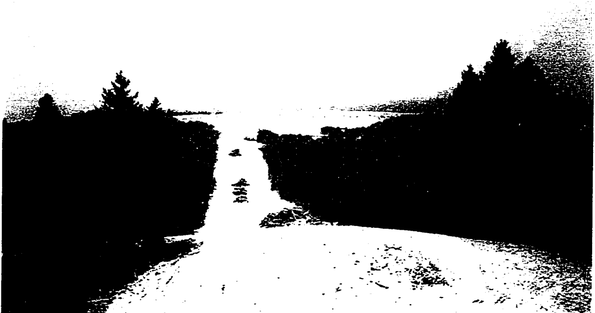
Figure 2.10: The full right-of-way stripping technique was used in treed areas (bushland). The entire twenty meter right-of-way is stripped in this technique.
