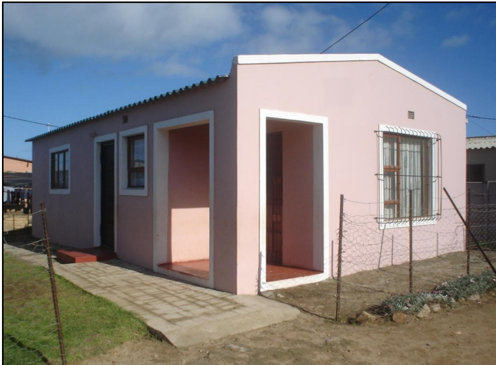
Figure 6.11: Extension (front portion) to original house (Photo credit: L. Roux)
