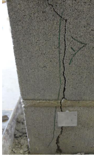
Wall 6-B (top splice)
