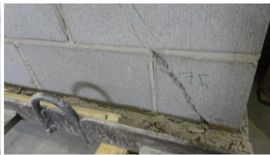
Wall 6-A (top splice)
