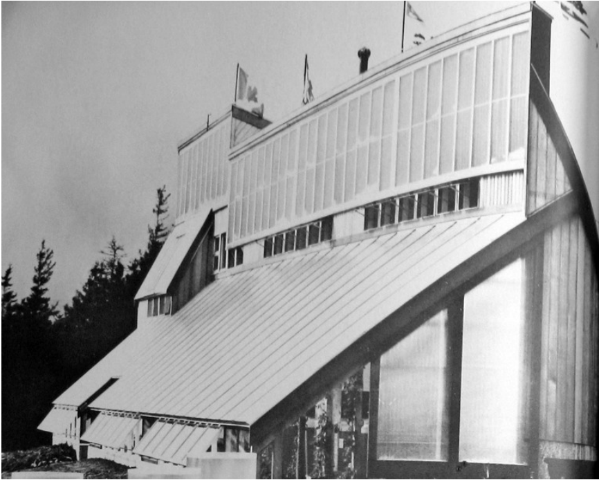
7.3 The PEI Ark viewed from the south. The greenhouse is in the right foreground and the living area in the left background. Source: An ARK for Prince Edward Island .
